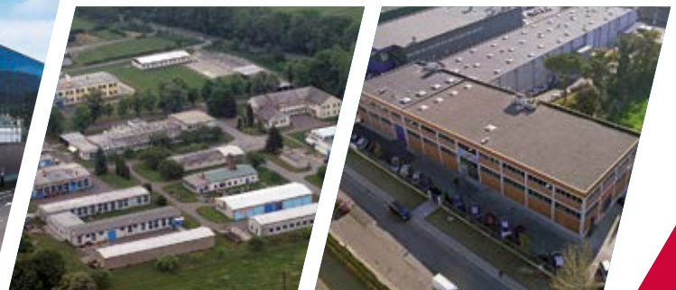
■ Two of the production centres of CIRCUTOR
